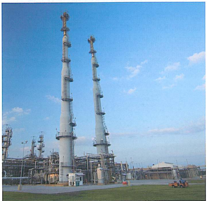
Thermal oxidizers located at ExxonMobil's Onshore Treating Facility in Theodore, Alabama.
